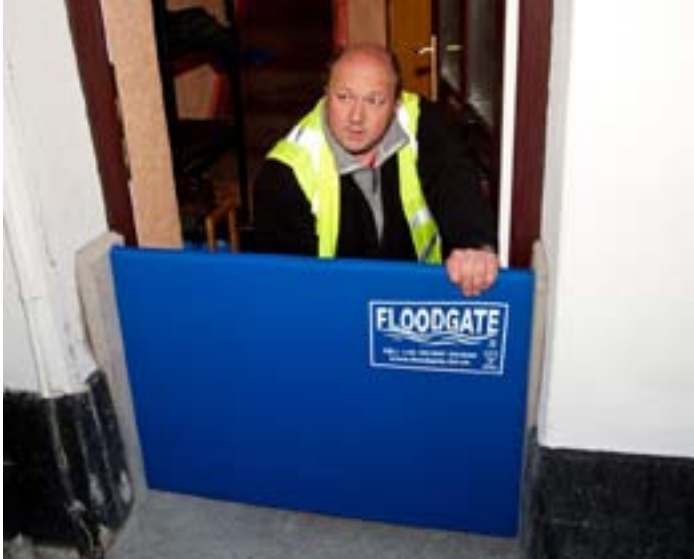
Andy White, of South Tawton Parsh Council, fitting a flood gate.
